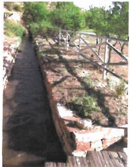
Rock constructed acequias located at a farm in Sena
