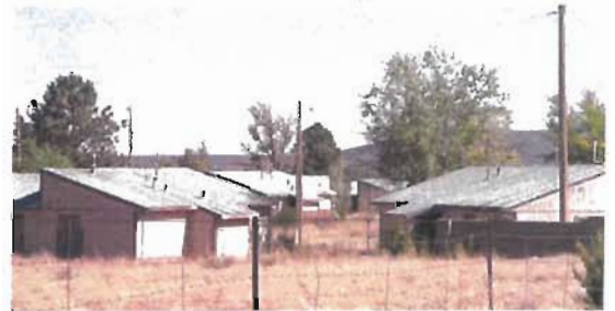
Old Ribera Public Housing. Location of the proposed San Miguel County redevelopment project.
